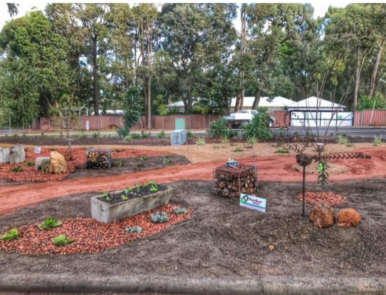
'Firewise' installation for the City of Armadale
