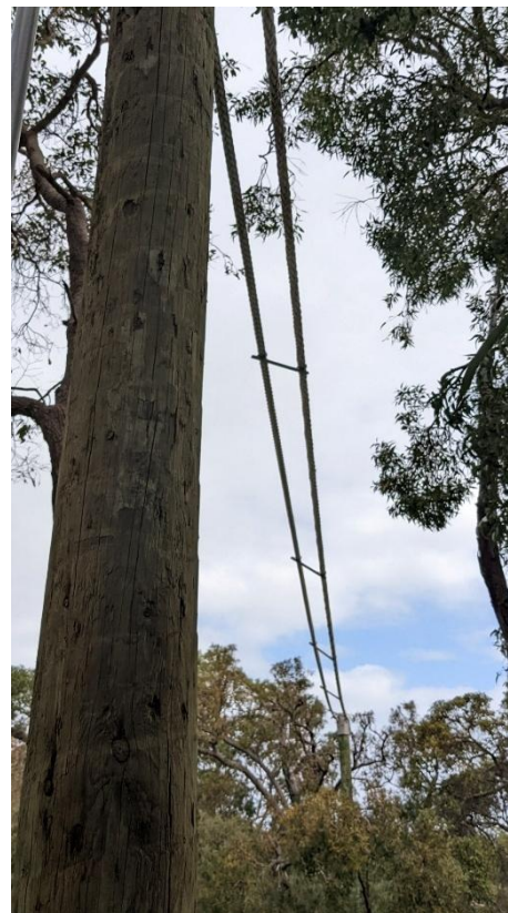
Figure 15: Possum Rope Bridge built to support Western Ringtail Possum movement through habitat retained within a residential subdivision in the City of Mandurah.
