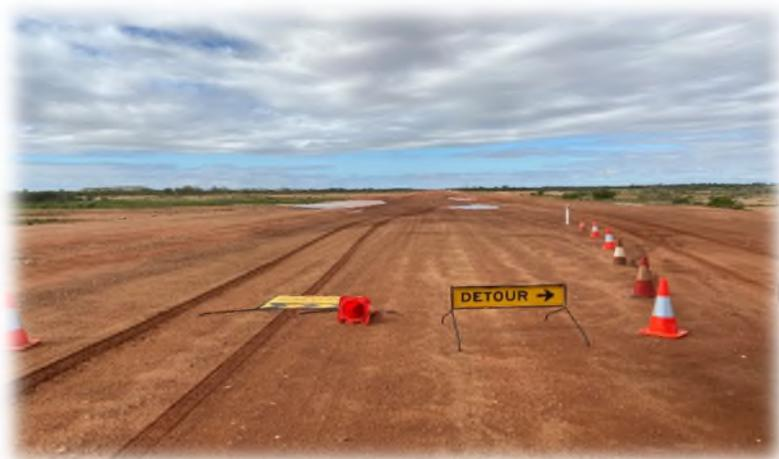
Figure 4: Road Closed sign run over and vehicle driving on works prepared for bitumen (\$1.3M)
