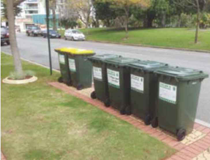
Figure 2: Hardstand bin pad adjacent to public roadway, provides a good example of a presentation point.
