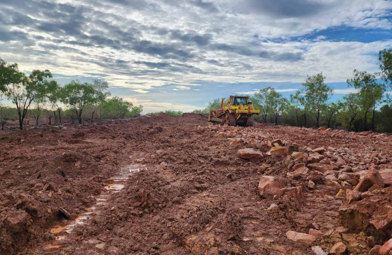
A Kimberley flood response dozer Credit: Main Roads
