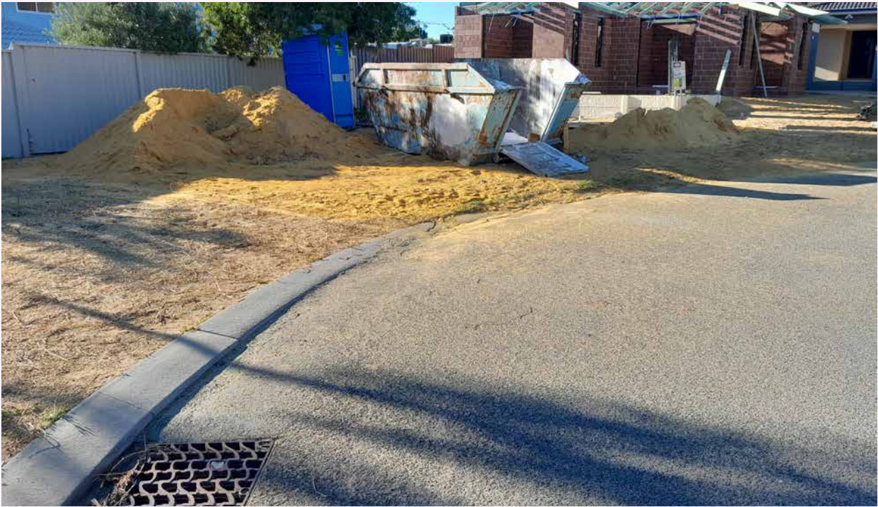
Sediment in the suburbs: This site could be improved by a sediment fence to capture sediment and prevent it from leaving the house block and simple additions such as tarpaulins to cover the sand piles, and a sediment sock around the drain to prevent sand from entering. Behaviour changes such as builders sweeping sand from the road at the end of the day would help too.
