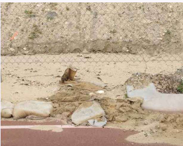
Left: Sand from the Mitchell Freeway extension leaving the site and blowing across the bike path.
