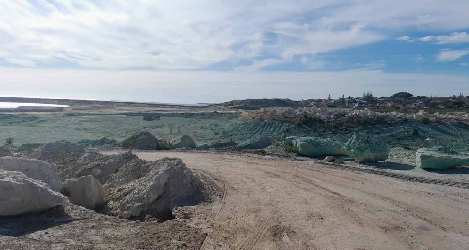
An example of excellent erosion and sediment control at the Development WA Ocean Reef Marina construction. The hydromulch (green in the photo) greatly reduces sand drift. NB: Photograph was taken over a sediment fence. Damaged silt curtain possibly causing sediment pollution near the site has been repaired.
