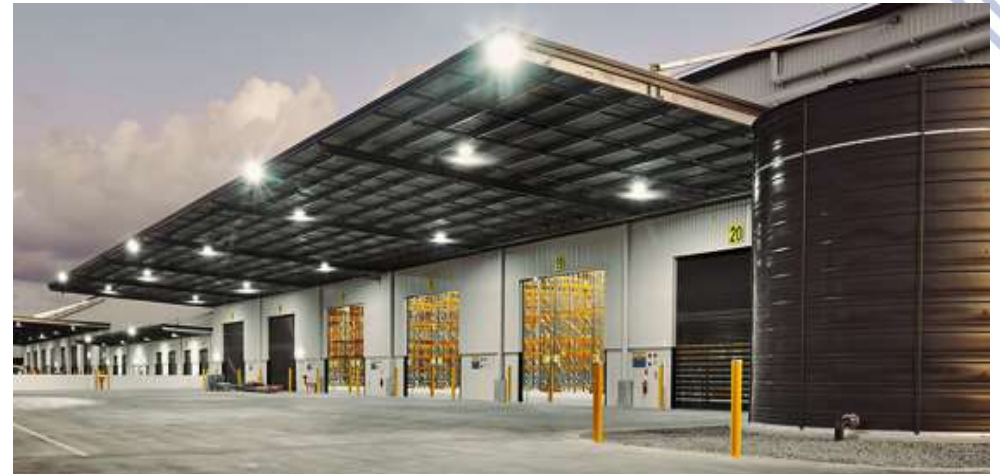
Figure 5: The Roe Highway Logistics Park has been recognised as Perth's most sustainable industrial site. Accessed online here on 22 February 2022.
